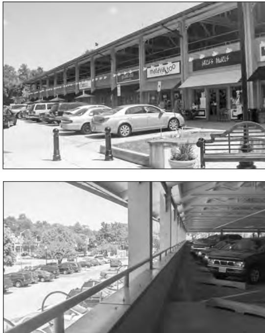
Example of a retail center with parking on the second level.
